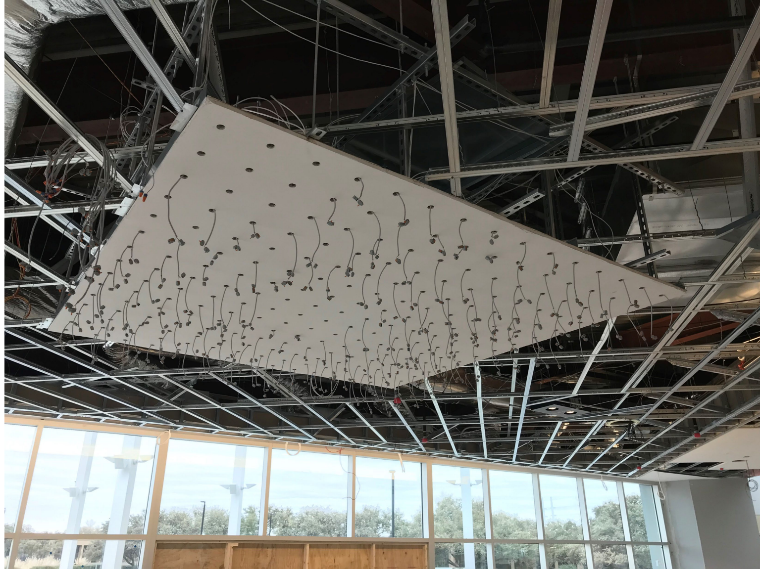
Lincoln Centre Dallas, Texas Custom Multispot Beluga with Trimless Mounting - Ceiling Preparation
